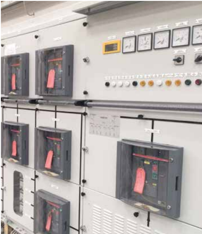
LV Main Switchboard 690V - 4000A - 85kA Internal Arc Execution
