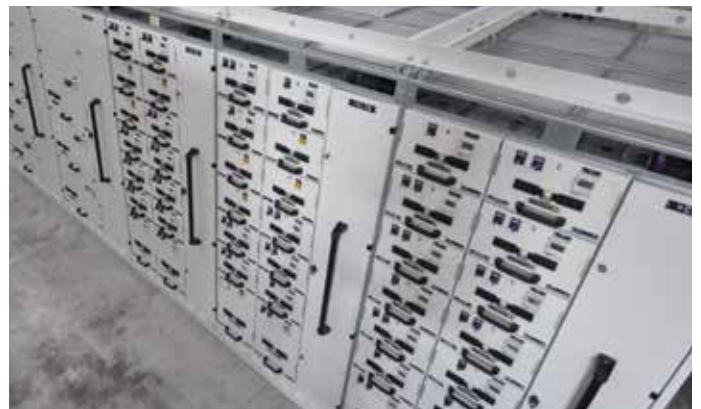
LV Main Switchboard 440V - 6300A - 80kA Internal Arc Execution
