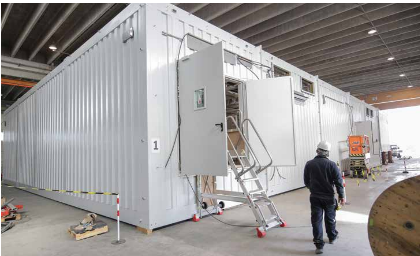
Surface approx 540 sq.m. Length Control Room assembled 28.5 mt; height 4.920 mt width 18 mt.
